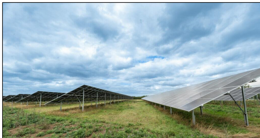
Figure 4 – Typical Solar Panel Mounting Structure
